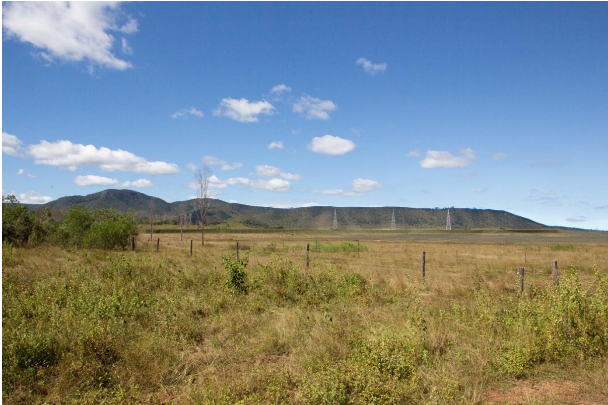
Figure 33: Location B, Image 2: Landscape with a grass berm hiding the batteries and substation. Upper sections of the three switchyard towers remain visible
