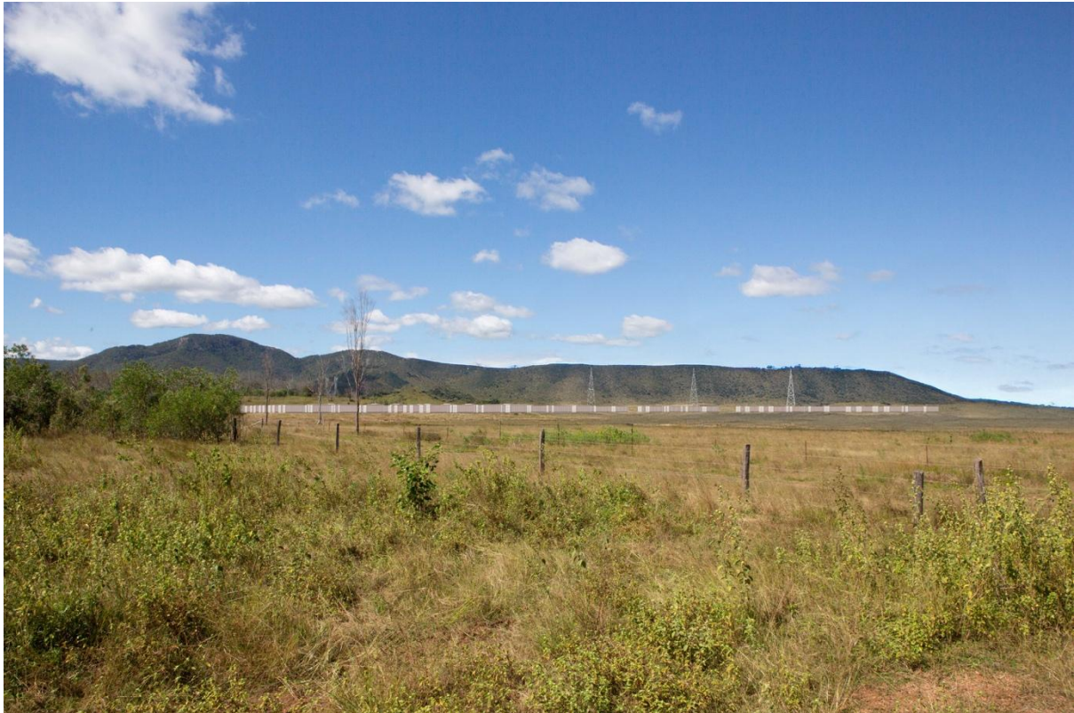
Figure 32: Location B, Image 1: Landscape with batteries and three switchyard towers visible
